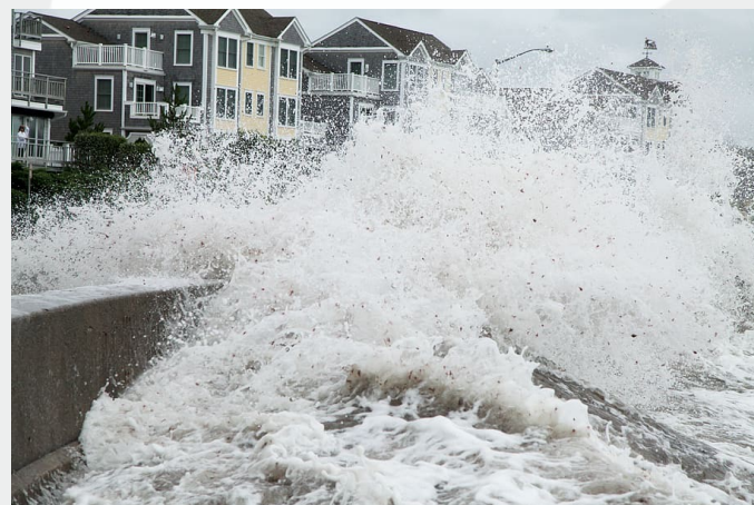
Storm Surge Kills
